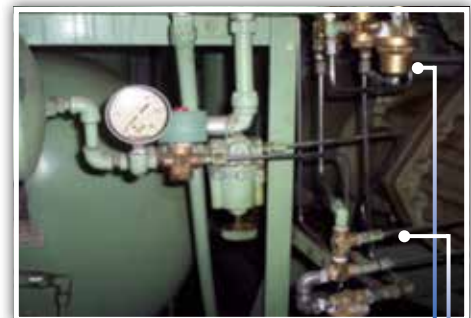
Spiral Valve Inlet Valve Differential
